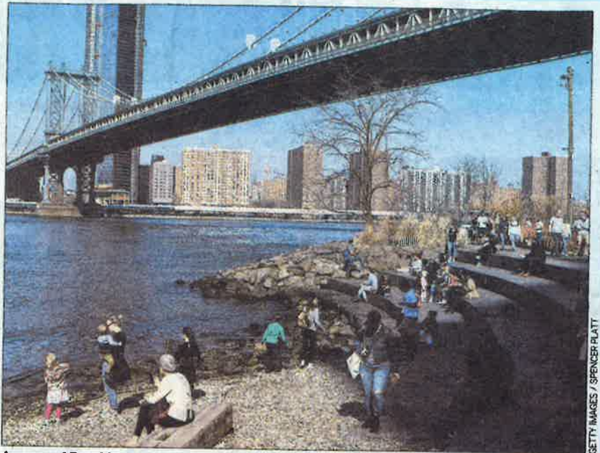
An area of Brooklyn Bridge Park will likely be closed until April due to falling debris.
